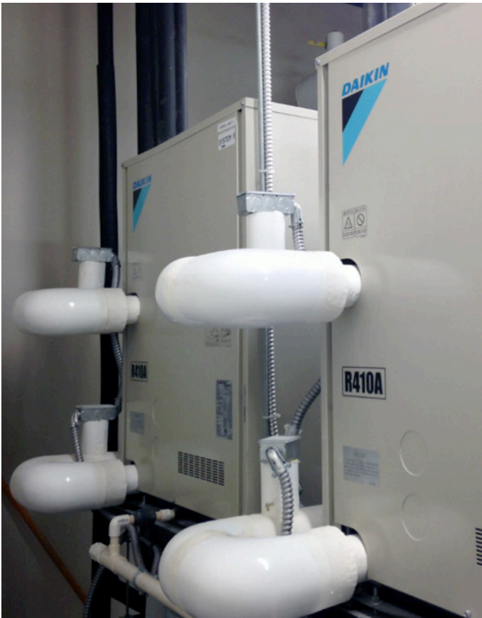
Figure 3. In a water-source VRF system, the condensing units (left) exchange heat with a fluid loop (white pipes); they distribute this energy to/from heat recovery controller (top right) which in turn distribute the energy to/from individual fan coil units at each zone (bottom right).
