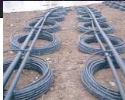
1. Heat exchangers being assembled on the shore of the pond. Each coil provides one ton of heating and cooling capacity.
